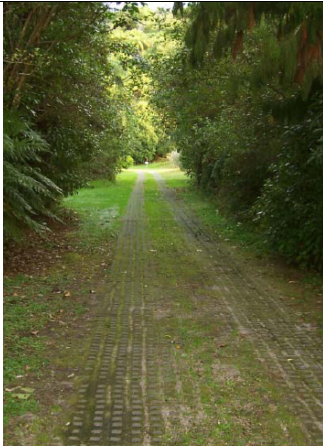
Figure 1 Photo of the porous carriageway at Haumingi 10a2b Papakainga
